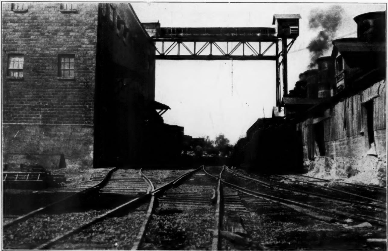
This Shows the Elevating and Conveying Unit from the Kilns at Right to the Hydrate Building at Left. Shipments Are Made by Rail from Either the Hydrate Plant or Kilns as Shown Here.
